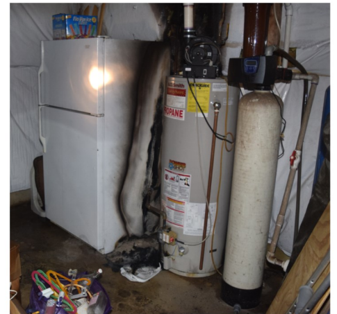
This fire was caused combustible material too close to the water heater and caused $5,000 in damages.
